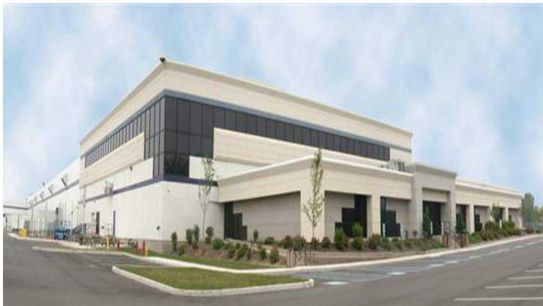
Figure 5-9 Typical Business in Liberty Industrial Park
