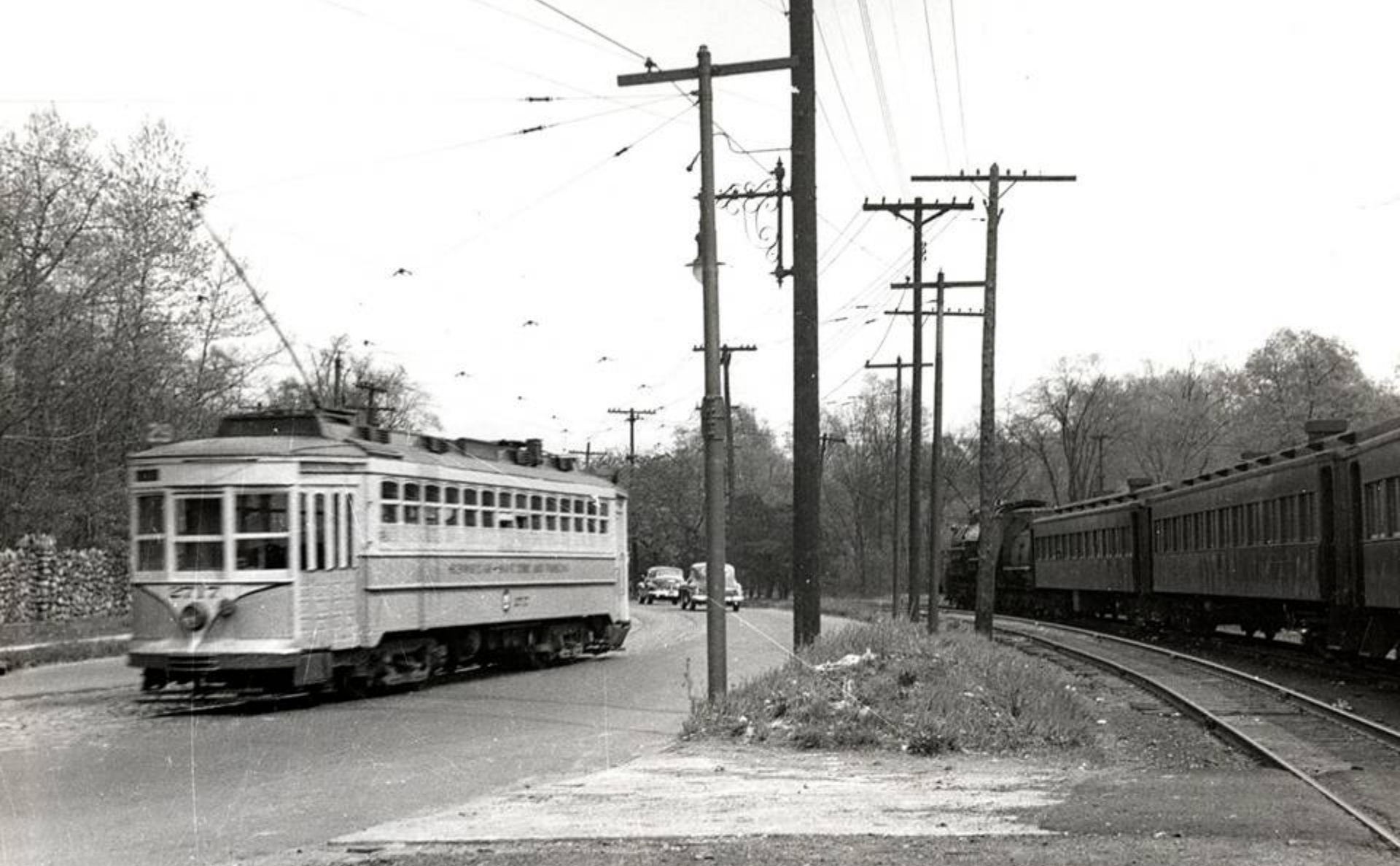
PSNJ 2717 Passing Erie RR on Bloomfield Ave. at Caldwell College (between Elm & Arlington) facing east. Stone wall at left is still there - but no traces of railroad (Erie Caldwell Branch-Morristown & Erie further south)--
