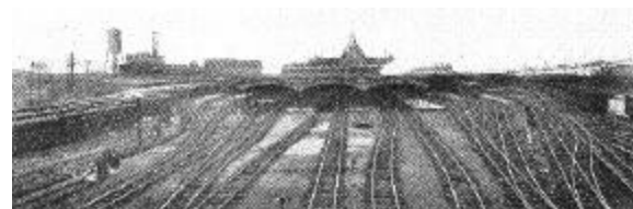
Figure 1.16: Shed under construction
