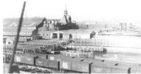
Figure 1.9: 1889 Train Shed and head house
