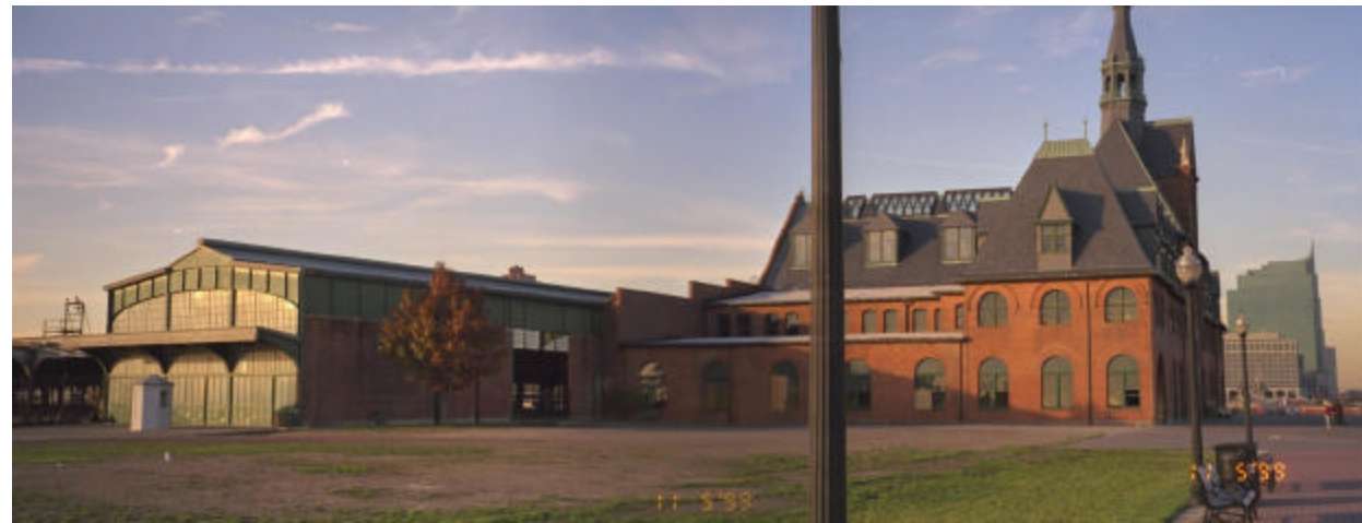
Figure 3.5: Head House and Concourse
