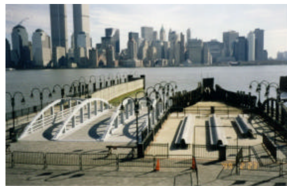
Figure 3.4: Ferry slip to the east of the Head House
