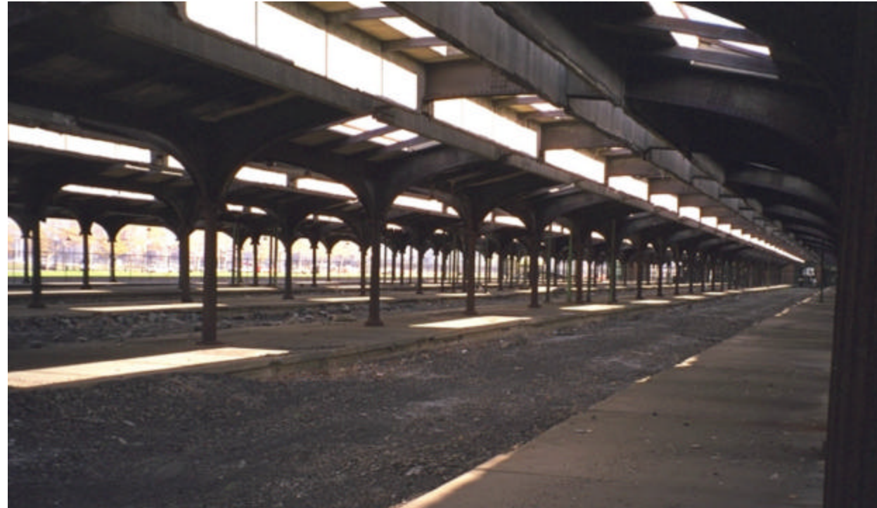
View of interior of the Shed
