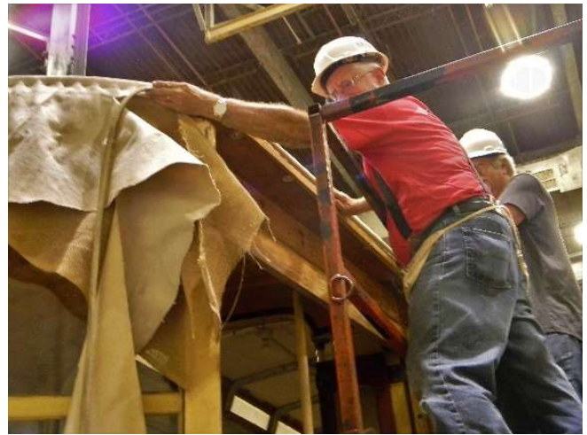
Time to trim the excess.
