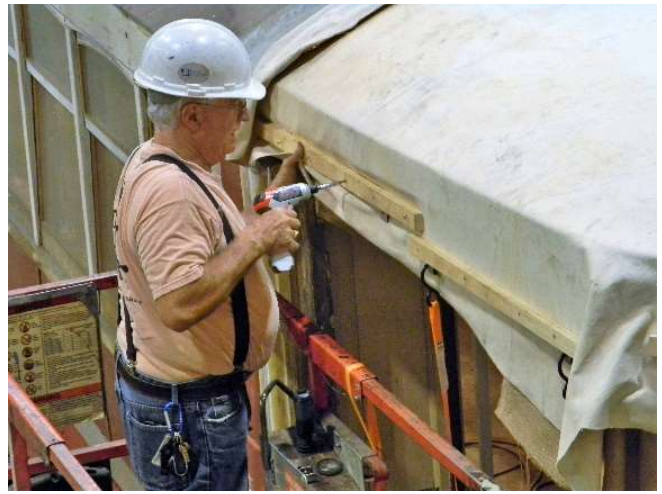
Jim attaches ratchet strap connector eyes to the grippers.
