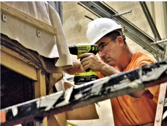
Teamwork rules the day as the connector eyes are attached and ever greater tension is applied to the canvas. Note: the bracket strap connector eyes, already in place (upper left).
