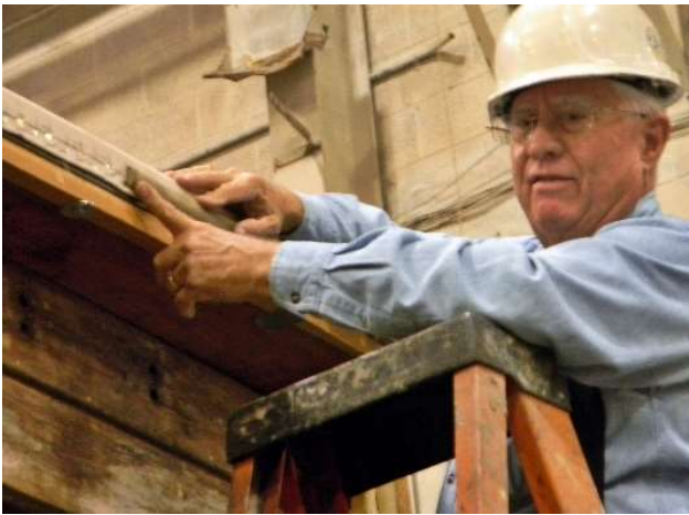
Jim places the plastic molding in preparation for pre-drilling and nailing.
