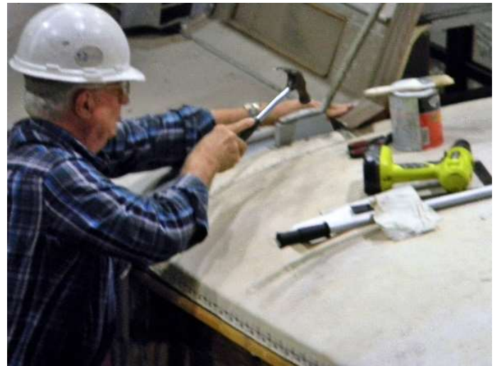
Nailing follows drilling.
