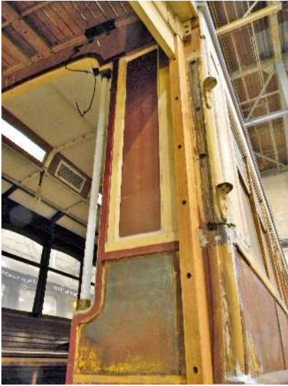
Bulkhead panels, removed in the P-Burg years by Hank Kaminski to facilitate structural repairs beneath, had to be refitted along with appertinent mitered quarter-round moldings.
