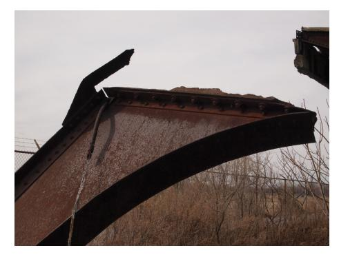
Former location of cantilever girder at A/14, showing remaining cast-iron column and top square-section connection extension, remaining A-line girders, and broken edges of cast iron
