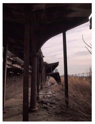
Concrete roof debris near A/15. Note the poor quality of the concrete at the broken edge and the spalled bottom.
